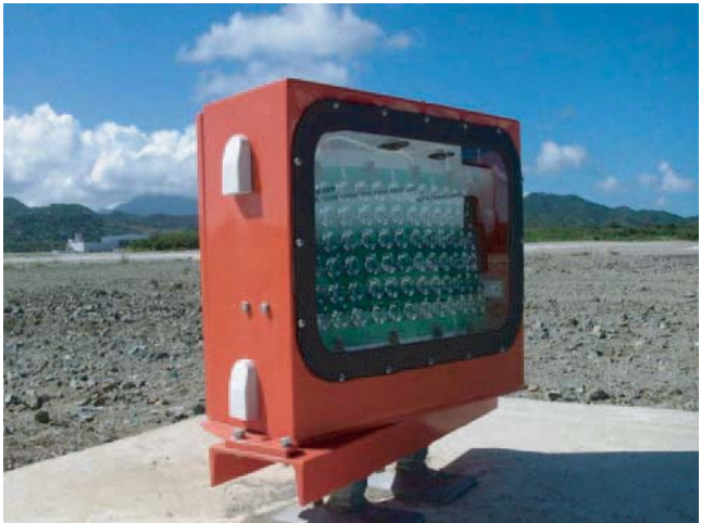
FIGURE 10 LED runway end identifier light.
