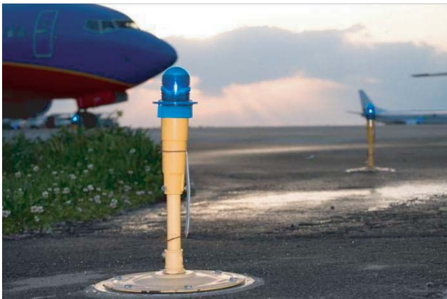
FIGURE 4 LED elevated taxiway edge light.
