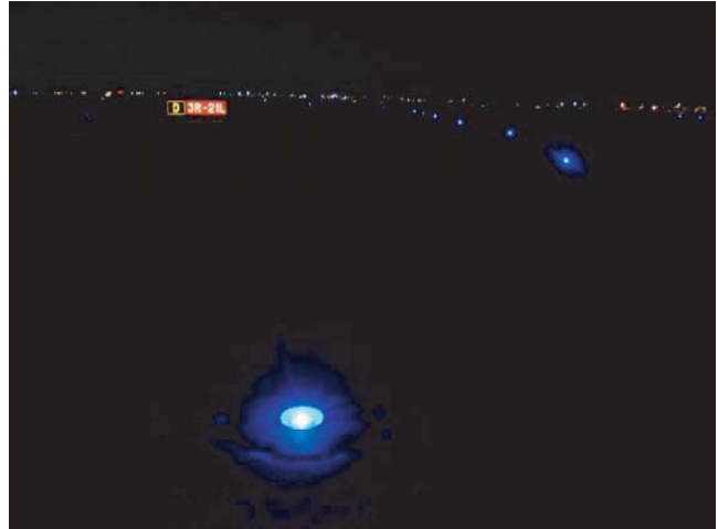
FIGURE 5 LED in-pavement taxiway edge light.
