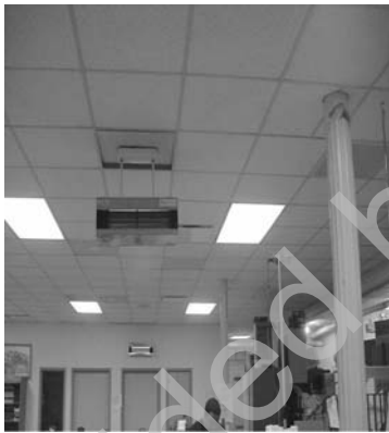
Fig. 13. Linear, instant start, germicidal lamps in UVGI pendant and wall mount fixtures. Source: TUSS Saint Vincent's Hospital, Manhattan, NY. Used with permission.
