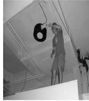
Fig.11. Cleaning and annual relamping UVGI pendant fixture. Source: TUSS Saint Vincent's Hospital, Manhattan, NY. Used with permission.
