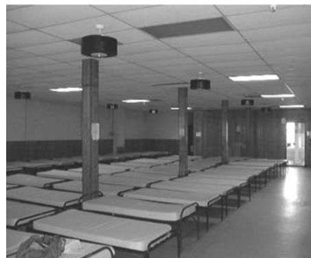
Fig. 16. Dormitory (congregate setting) using pendant mounted (compact) germicidal fixtures delivering UVGI in 360°. Source: TUSS Saint Vincent's Hospital, Manhattan, NY. Used with permission.
