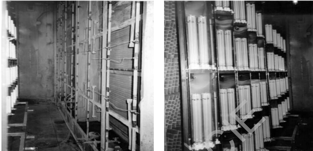
Fig. 20. In duct air irradiation (Lumalier™ ExStream system) designed for installation at the Willard Hotel Complex, Washington, DC. Disinfecting over 30 000 m 3 /min and 8 m (25-foot) cooling coil. Source: Lumalier Inc. Used with permission.
