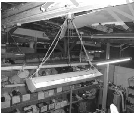
Fig. 15. Suspended UVGI fixture for high bay (> 3 m floor to ceiling height) application. Uses compact germicidal lamps. Source: TUSS Saint Vincent's Hospital, Manhattan, NY. Used with permission.
