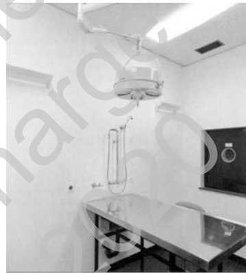
Fig. 14. UVGI fixtures directing energy upward and downward in a laboratory application to reduce infectious organisms. WARNING: Workers in this setting must wear protective gowns and goggles to protect all exposed eye and skin surfaces from over exposure to UV-C. Source: Philips Lighting. Used with permission.
