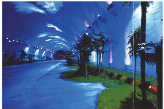
Figure 20 Examples of architectural measures to counteract monotony and fear from the Lærdalstunnel in Norway and the Zhongnanshan tunnel in China (Photo: SINTEF, with kind permission).
